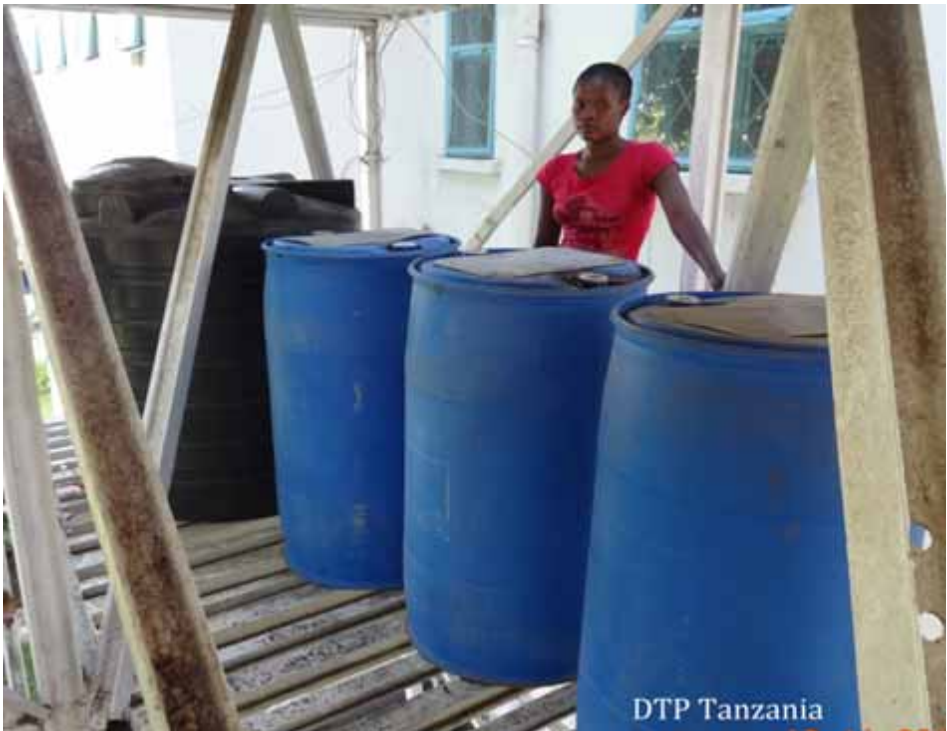
Figure 9. A triple filtration plant based on bone char installed at an international school in Arusha.
