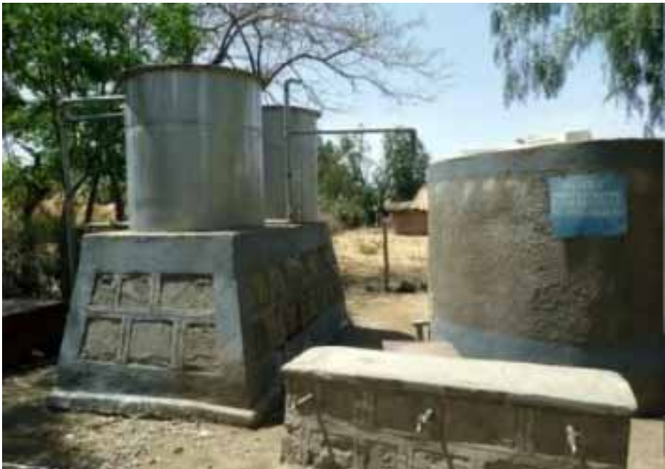
Figure 11. The domestic defluoridation filter, based on bone char, of the Catholic Diocese of Nakuru, CDN.
