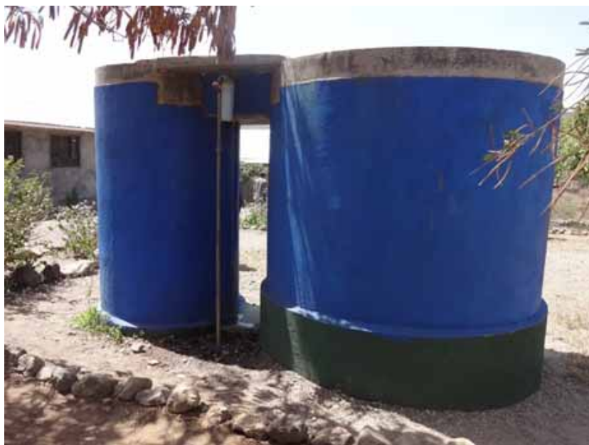
Figure 10. A defluoridation plant built by the Ministry of Water in Tanzania for bone char defluoridation at a village school.
