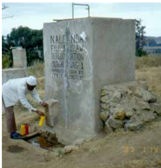
Figure 4. The DTP-fill and draw defluoridation plant at Oldonyowasi based on the Nalgonda technique.
