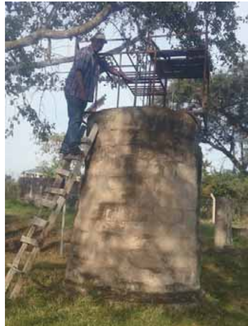
Figure 5. The Nalgonda technique community defluoridation plant developed by the Ministry of Water in Tanzania. 28
